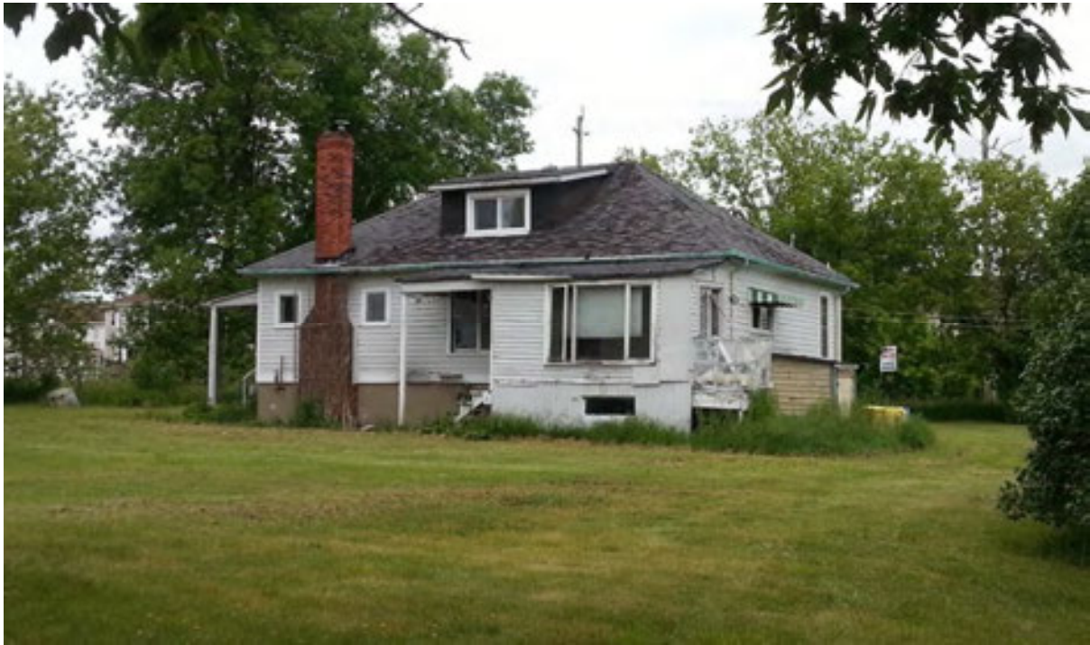
Photo 11: Looking north at the rear of the residence located at 612 John Counter Boulevard. Fill and vent pipes can be seen on the left side of the house.
