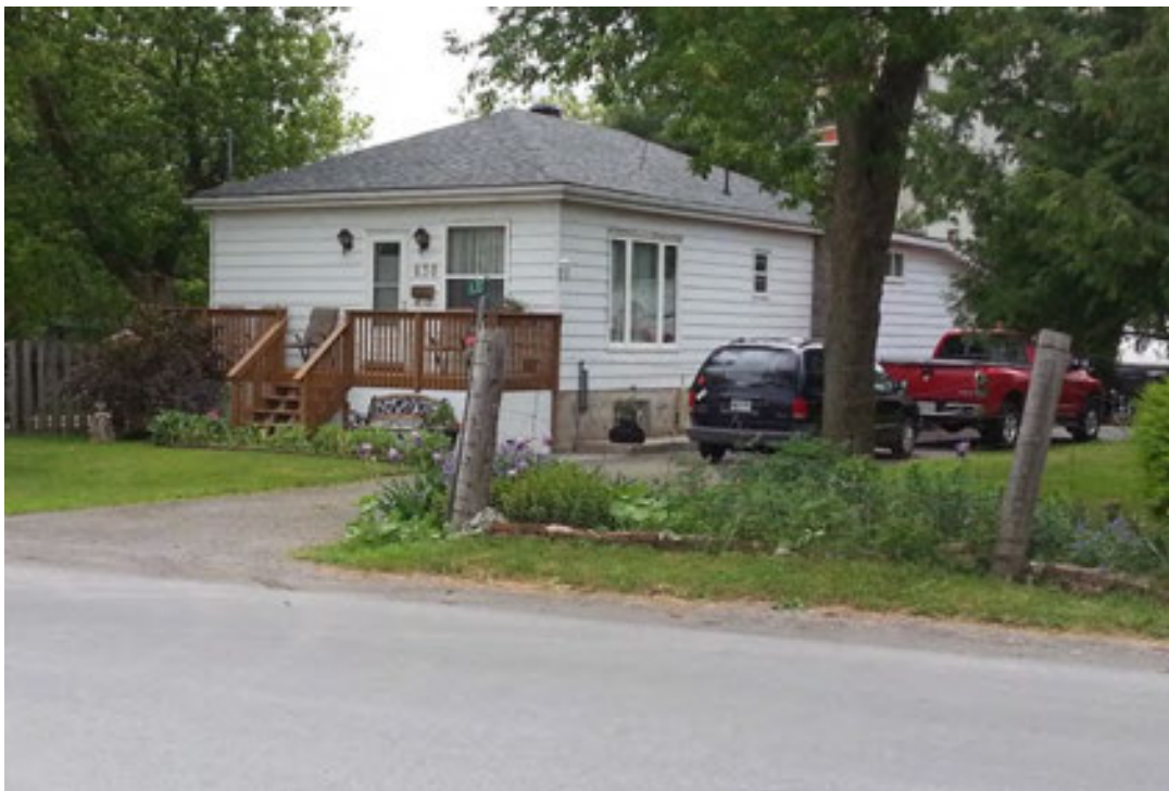
Photo 10: Looking south at the residence located at 630 John Counter Boulevard. Vent and fill pipes can be seen on the corner of the house to the right of the front porch.
